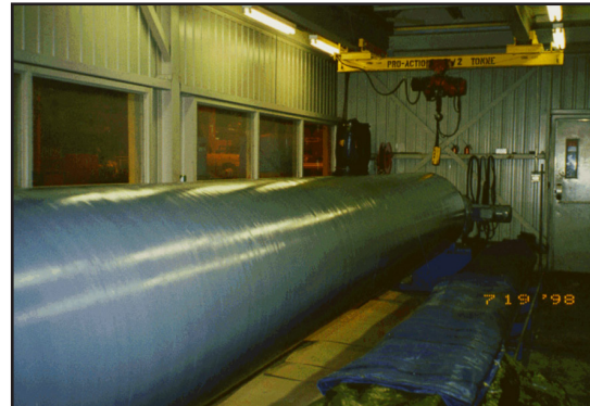
ARC 858 being applied
